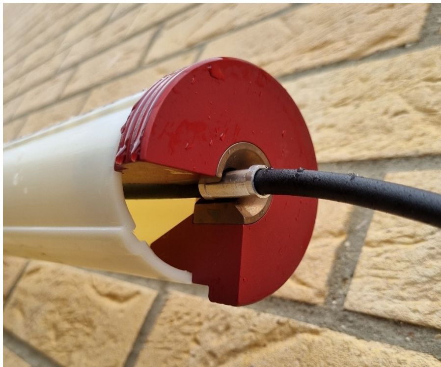
Figure 24: Cable gate fitted onto the access end of the casing
