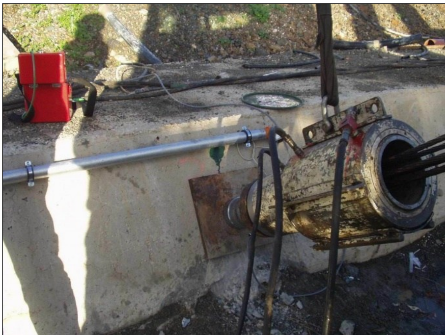
Figure 9: Jack placed above load cell
