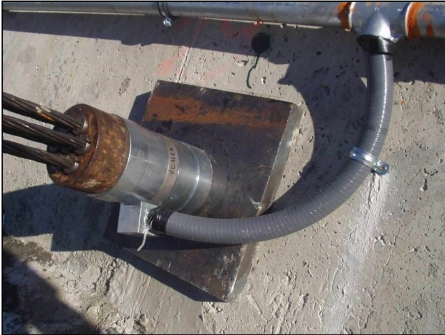
Figure 8: Bearing plate fabricated and placed between wall and loadcell distribution plate
